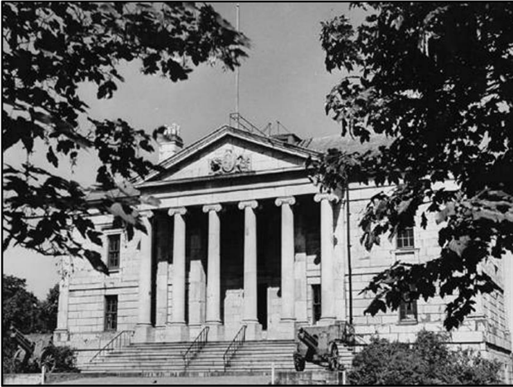
Colonial Building, St. John's, seat of Newfoundland House of Assembly (1850-1933, 1949-59) and locale of National Convention 1946-48. Built in 1850 of neoclassical design fronted by Irish limestone with six ionic columns and pediment sculpted with royal coat of arms
